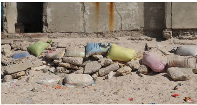
Figure 4: Protection of coastal region with sand bags.
