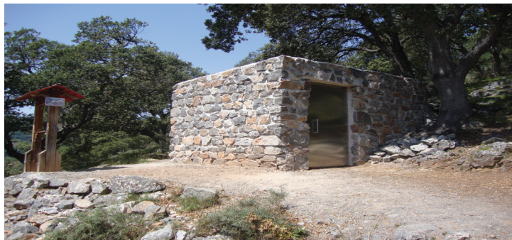
Figure 4) Old entrance door and new climate access camera
